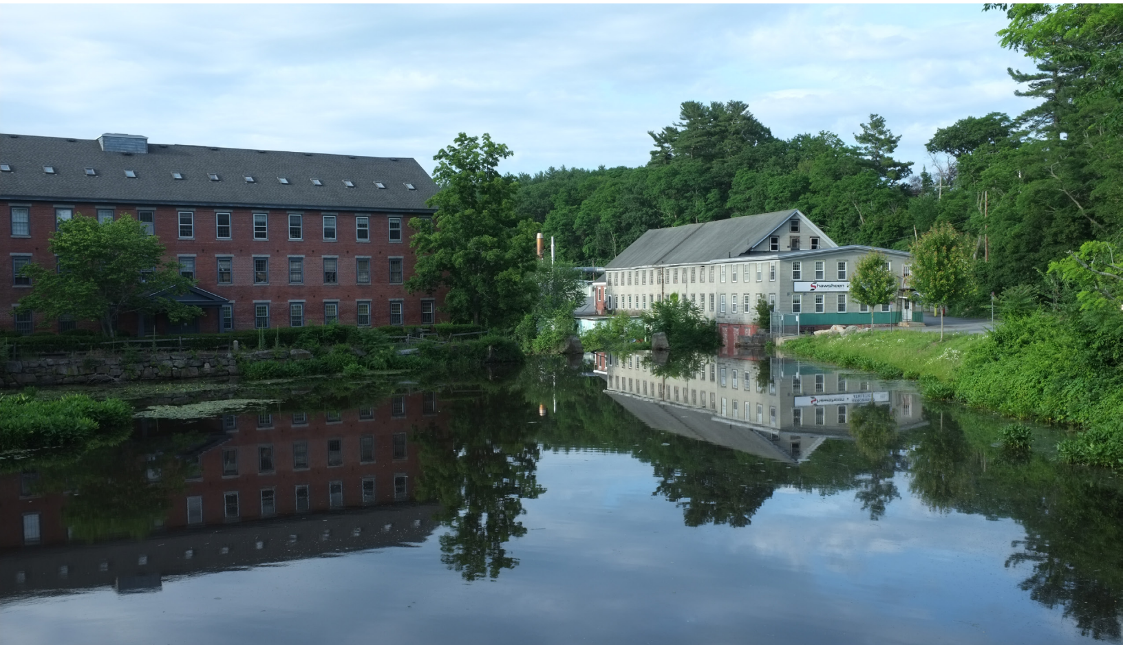
Ballardvale Dam on The Shawsheen River. June 23, 2023. Photo by Jon Unger
